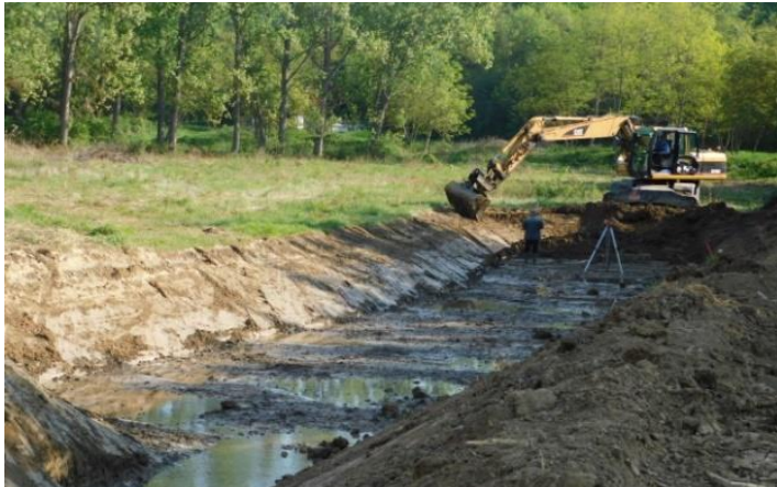
26 – Works in progress in Püspökszilágy. (Photo: the Municipality of Püspökszilágy)
