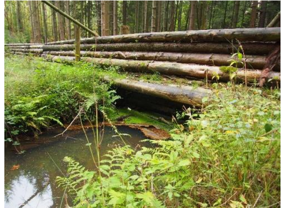
6 – Leaky log dam in the forest above Pickering, England. (Photo: Klára Kerpely, WWF HU)
