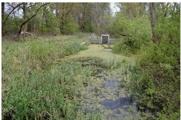
8 – A section of a canal transformed and managed for water retention in the region called Turjánvidék. (Photo: Annamária Csóka, http://turjanvidek.hu/ )
