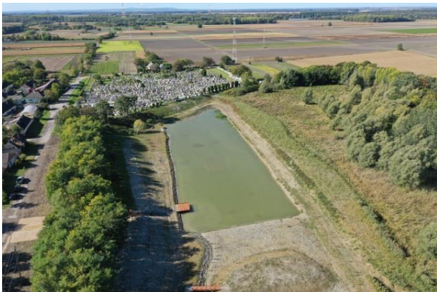
23 – The finished project: two-basin open-surface reservoir pond. (Photo: Filmever Stúdió)
