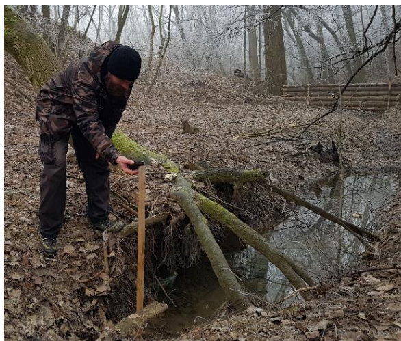
48 – A simple measuring system to monitor how the storage basins above the log dams installed in the erosion gully are silting up. (Photo: WWF HU.)
