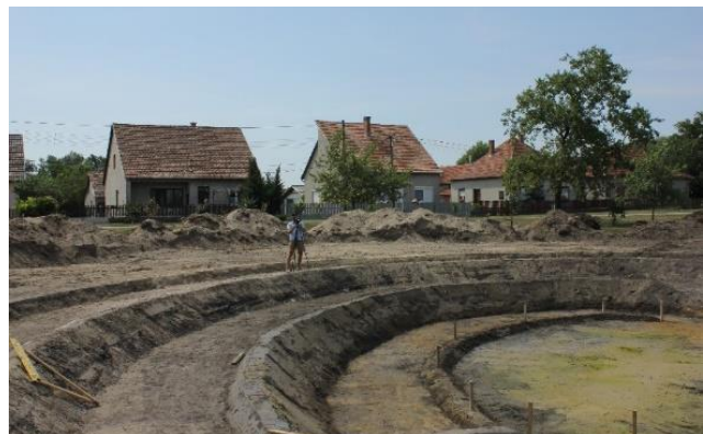
32 – Shaping a varied lake bed surface for the local pond at Ruzsa. (Photo: WWF HU.)
