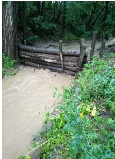
28 – Log dams at Püspökszilágy during the dry period, and “at work”. (Photo: Ministry of Interior, Püspökszilágy Municipality)
