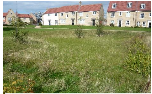
11 – Storm water reservoir suitable for temporary inundation, also functioning as a green surface. (Source: susdrain.org)
