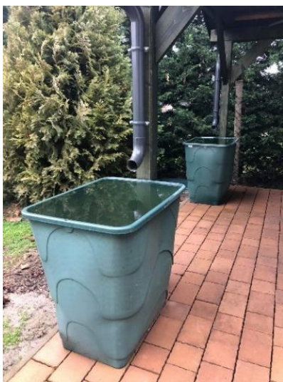
13 – A simple and inexpensive rainwater collecting system for retaining and utilising rainwater around the house. (Photo: Zsófia Szabó, Bátya)
