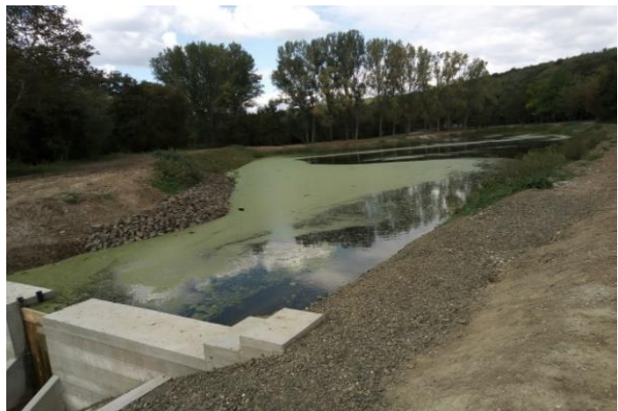
27 – Construction operations in progress in Püspökszilágy. (Photo: The Municipality of Püspökszilágy)
