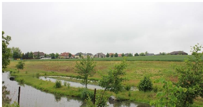
2 – In the Czech village of Hostovice the risk of flood was reduced by restoring the bends of the stream flowing through the village and by flattening its floodplain, creating an attractive park in place of a former canal. (Photo: Viktor Mátyás Farkas, WWF HU)
