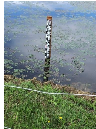
42 – Installed water level gauge at Tiszatarján. (Photo: the Municipality of Tiszatarján)
